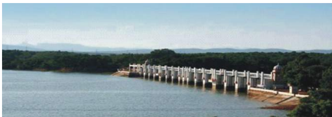
Overview of the Reservoir
